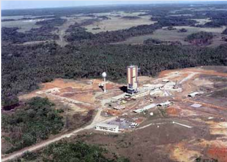
ELA 1 en construction
