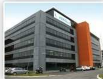
HQ & Engineering center
